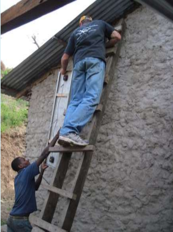
Left: Installing the solar panel on the back side of the roof.
